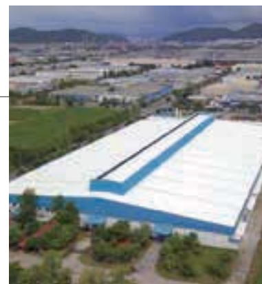
Fujitsu General (Thailand) Co., Ltd. (Thailand) FACTORY-2
