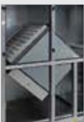
Heat recovery Cross flow type
