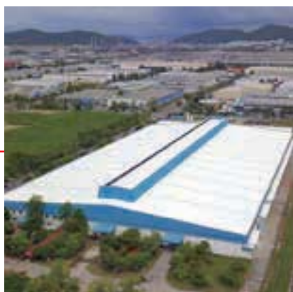
Fujitsu General (Thailand) Co., Ltd. (Thailand) FACTORY-2
