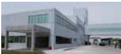
R&D Center in Fujitsu General (Shanghai)
