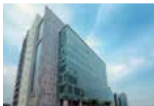
ABS Aircon Engineers Private Ltd. (India)
